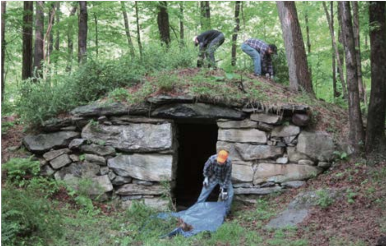
Maintenance work on a corbelled stone chamber. Photo © Beth Herr.
