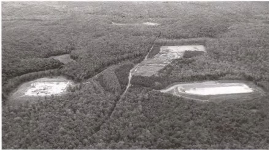
Fortuna Energy site (tract 587) in Tioga State Forest, PA, illustrating degree of forest fragmentation of a single HVHFF installation. Photo: Dick Martin of www.PAForestCoalition.org .
