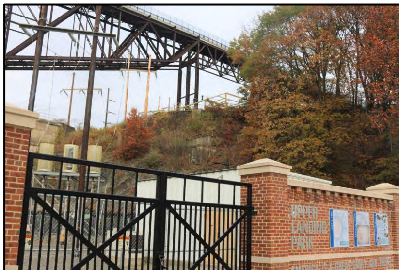
Example of mix-use of Hudson River shoreline: utility space, habitat space and public access space (foreground to background). E. Heffernan © 2018
