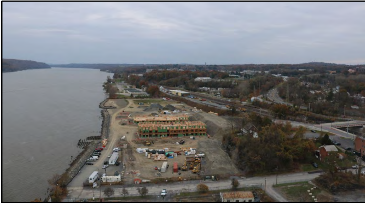
New construction along northern shore of Hudson River. E. Heffernan © 2018
